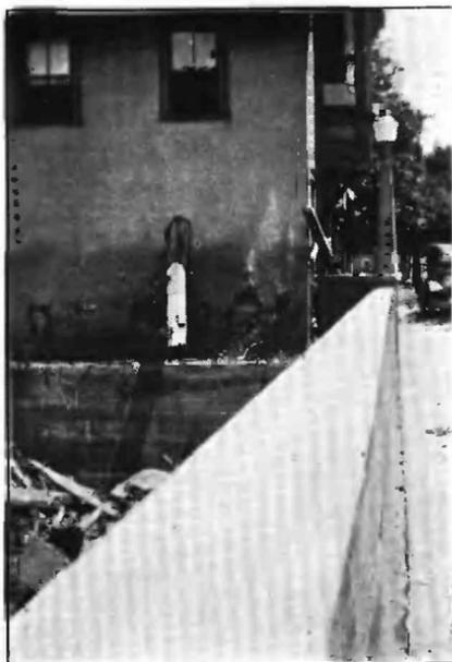
B. TELEPHONE POLE DRIVEN THROUGH SIDE WALL AND CEILING INTO THE SECOND FLOOR OF A HOME ON RIVER STREET, HORNELL, N. Y.
