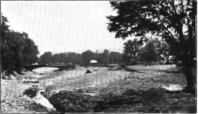
A. TAUGHANNOCK FALLS STATE PARK, N. Y., SHOWING DESTRUCTION OF ROAD DUE TO INADEQUACY OF BRIDGE TO CARRY FLOOD WATERS.
