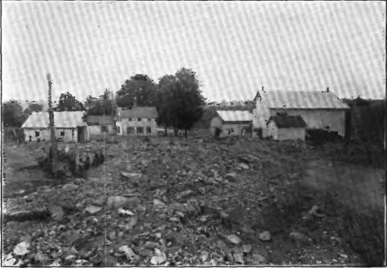
A. CHARLES BECKWITH FARM, SOUTH OF OXFORD, N. Y., SHOWING TYPICAL DAMAGE BY STONES AND GRAVEL TRANSPORTED BY SMALL STREAMS.
