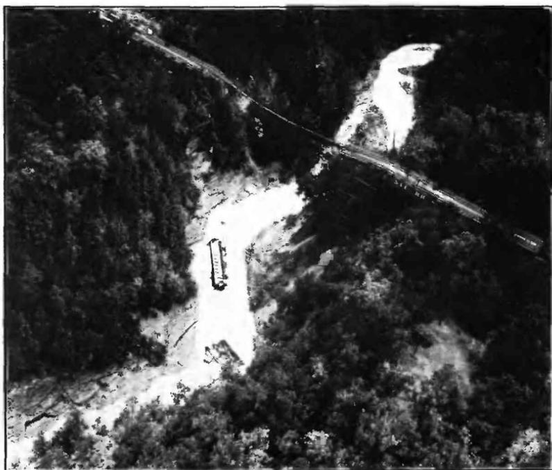
**B. NEW YORK CENTRAL RAILROAD AT WATKINS GLEN, N. Y., SHOWING HIGH BRIDGE OVER GLEN CREEK DESTROYED DURING THE FLOOD.**
