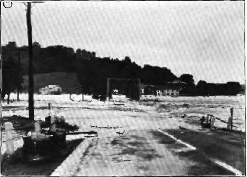
A. CHENANGO FORKS, N. Y., AT JUNCTION OF TIOUGHNIOGA AND CHENANGO RIVERS, SHOWING INADEQUACY OF BRIDGE OVER TIOUGHNIOGA RIVER TO CARRY FLOOD WATERS.
